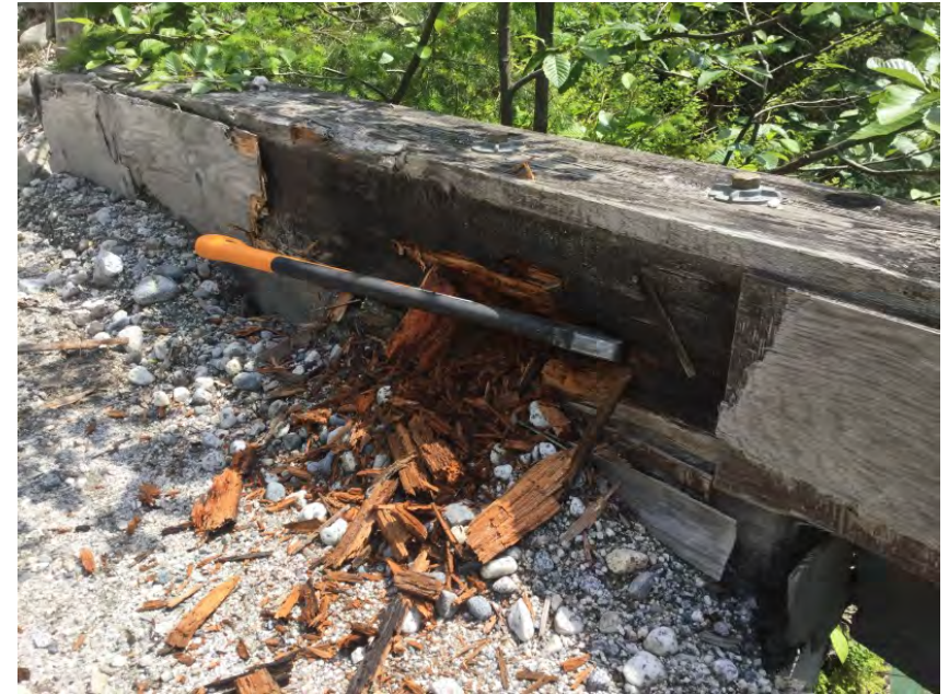
Guardrail condition at left approach
