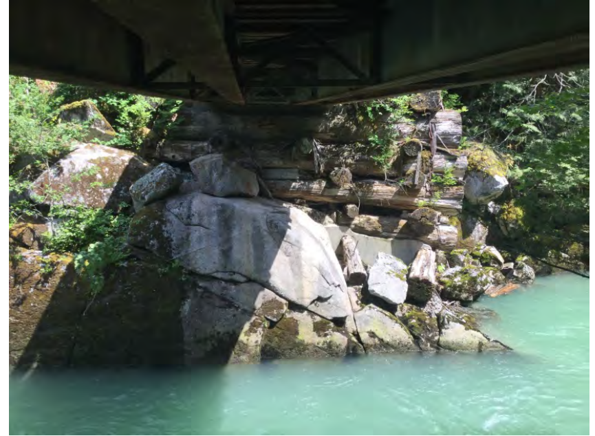
Left Bank Abutment when facing downstream
