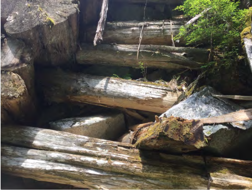
Downstream left wingwall
