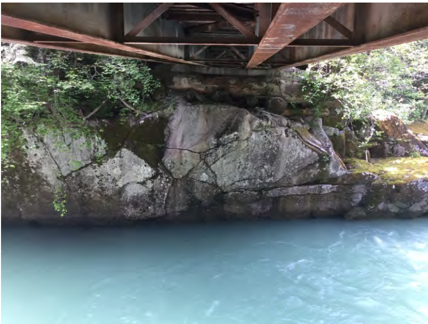
Right Bank Abutment when facing downstream
