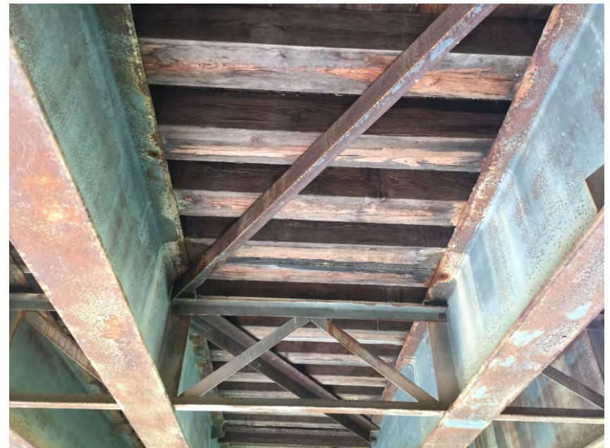
Deck from underneath
